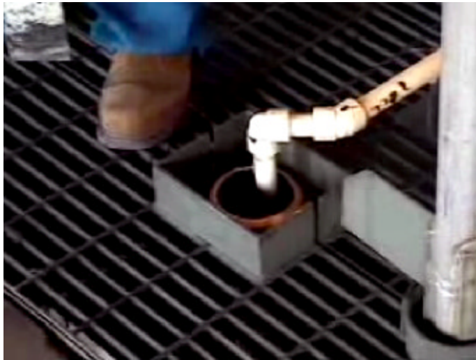
Visual image of open-ended drain
